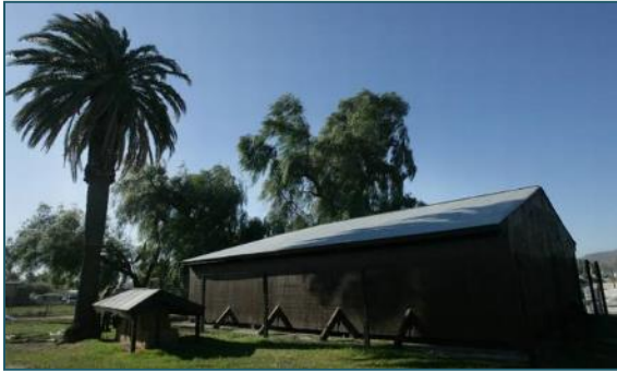
Structure built to preserve the Trujillo Adobe
