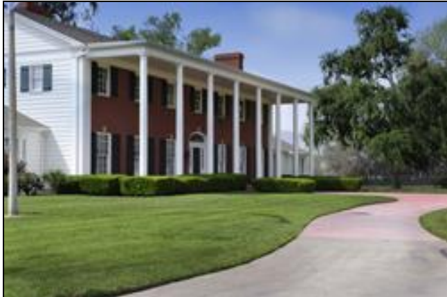
Crestmore Manor Facade
