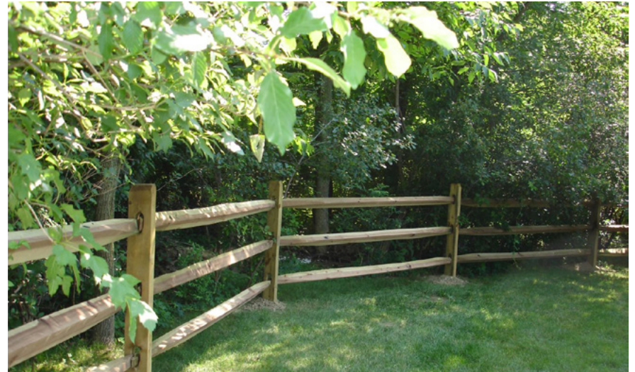
Low Security Fencing
