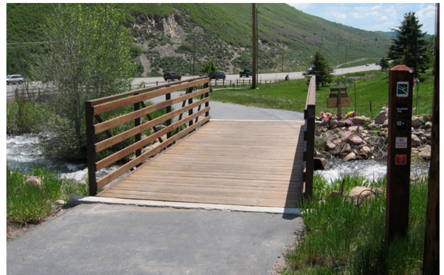
Wood and Cor-Ten Steel Bridge - Millennium Trail (Park City, UT)
