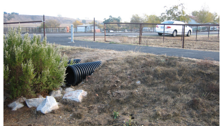
Culvert (Atascadero, CA)
