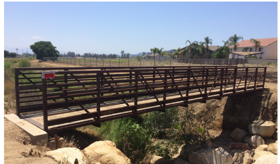
Prefabricated Steel Truss Bridge - Murrieta Creek Trail (Wildomar, CA)
