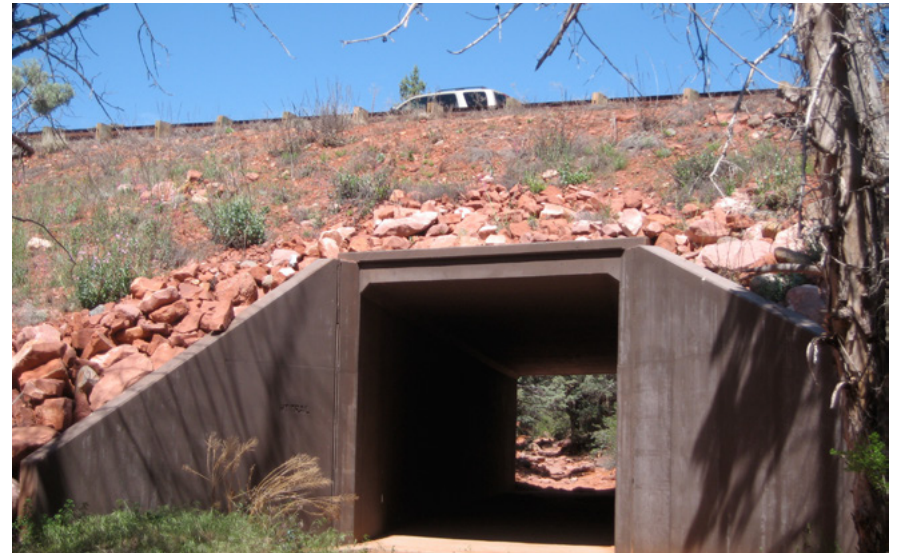
Highway Underpass - HT Trail (Sedona, AZ)
