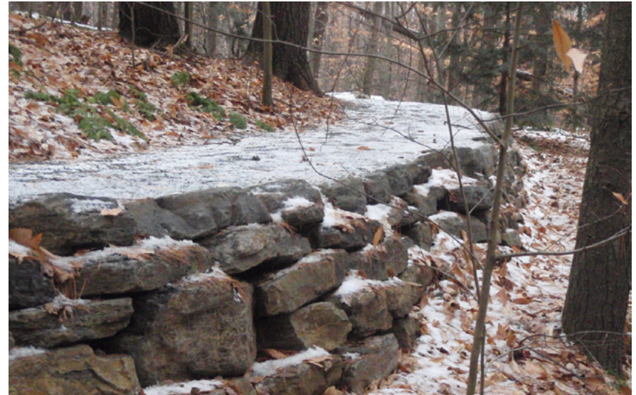
Stone Retaining Wall - Upper Valley Trail (Quechee, VT)
