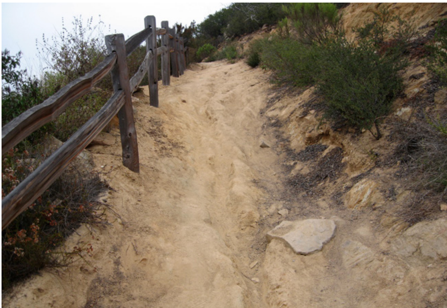
Examples of Excessively Steep Trails Suffering from Recurring Erosion and Widening as Users Move Outward to Avoid Ruts
